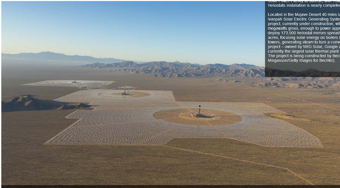
Solar Power Facility at sunrise, with tower. Heliostats installation is nearly completed.
